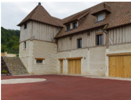
View of the backyard with turret.
