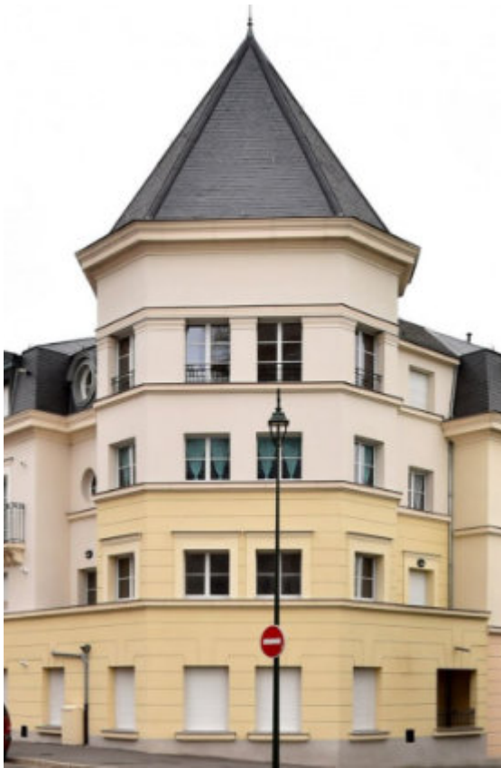
Above - A hexagonal corner tower, opposite the town hall [1].
